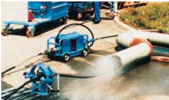
Internal pipe cleaning with high-pressure water jet RDR-system
