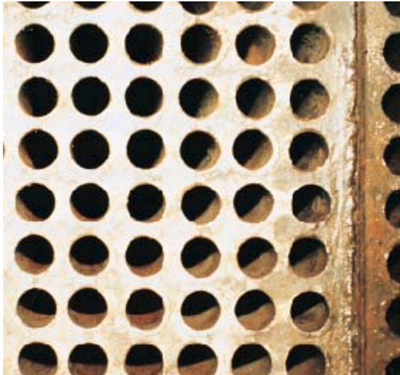
Heat exchanger cleaned by high-pressure water jetting
