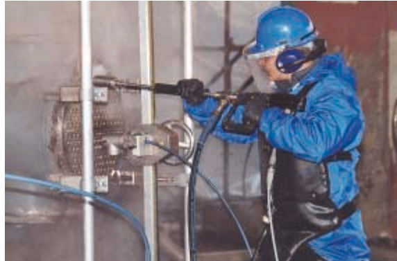
Surface cleaning with hot water gun and OrbiMaster®
