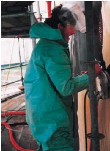
Emission-free paint stripping from tanks
