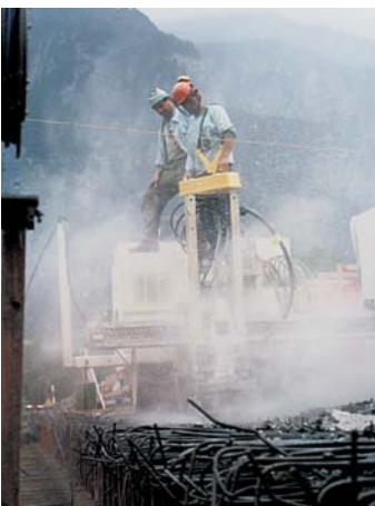
Exposing reinforcement bars
