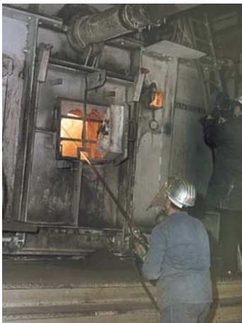
Cleaning of cement kilns
