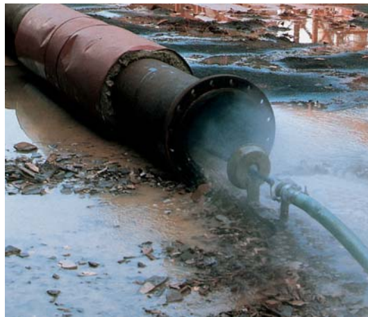
Internal cleaning of pipes
