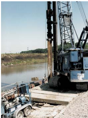
Water jet assisted pile driving
