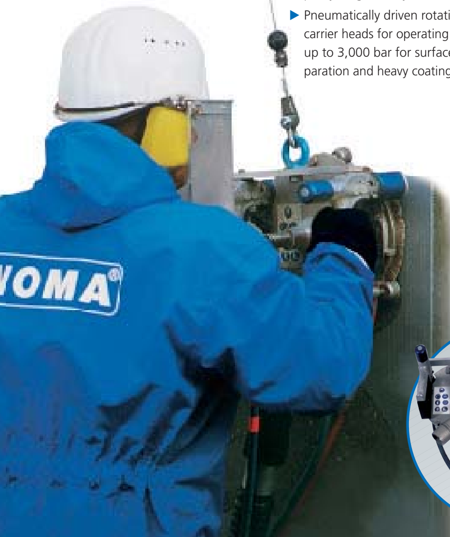
Ultra-high pressure water jetting tool type Eco Top Rotating Cleaner for emission-free surface preparation
