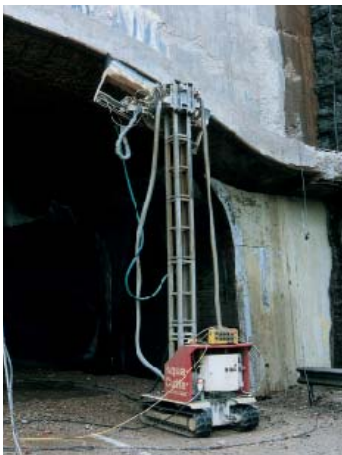
Selective removal of concrete
