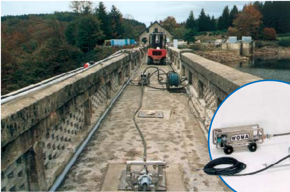
Pneumatically driven high-pressure water jetting tool type TubeMaster® for internal pipe cleaning
