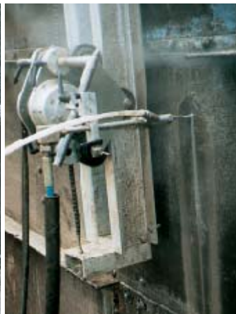
Demolition of vessels
