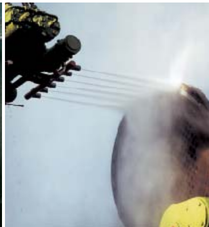
Cleaning of tube bundles
