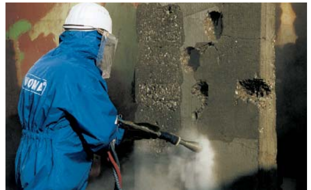
High-pressure gun with pneumatically driven rotary lead-through type Speedy 3000 and rotating nozzle carrier head type E 09 for concrete de-coating
