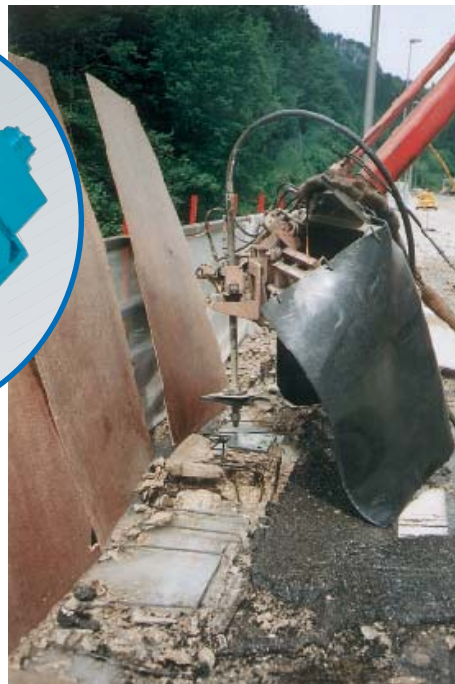
Hydraulically driven high-pressure water jetting tool type Orbiter for concrete hydrodemolition
